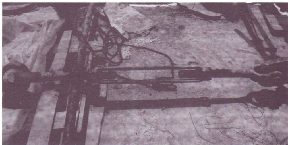
Figure 9. CROSBY turnbuckle type HG-228 for sag removal.
