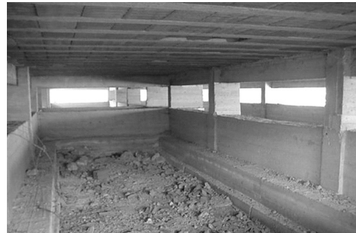
Figure 2. Partial view of foundation.
