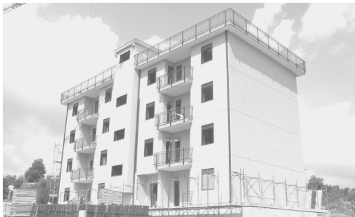
Figure 21. View of the tested Solarino building.
