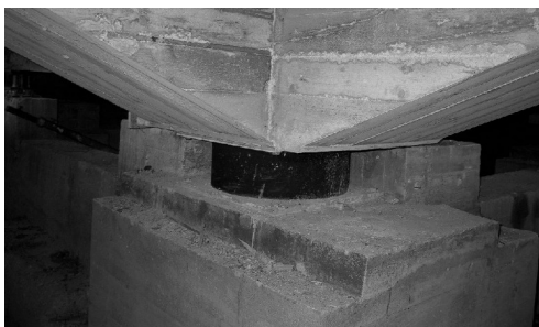
Figure 6. High Damping Rubber Bearing.
