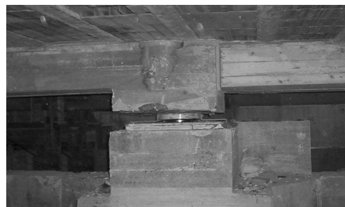
Figure 7. Low Friction Sliding Bearing.
